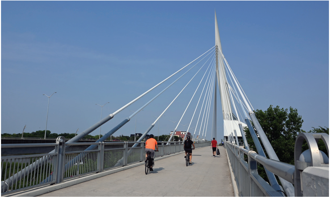
St. Boniface walking bridge / Alanna Yuen
