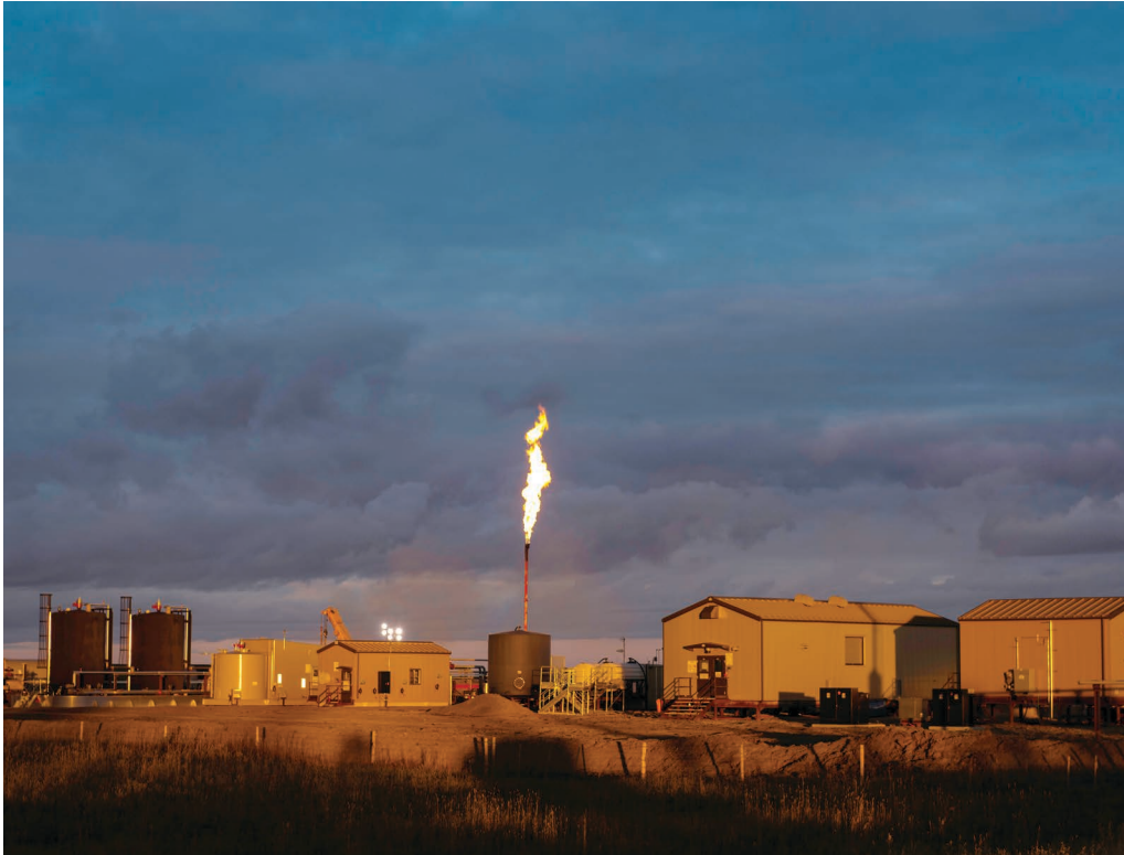
NATURAL GAS FLARING NEAR TOWER GAS PLANT. PHOTO BY GARTH LENZ.
